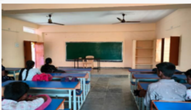
After classroom repair with tandoor tiles
