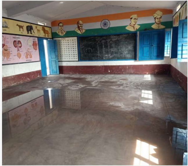
Flooring at community hall
