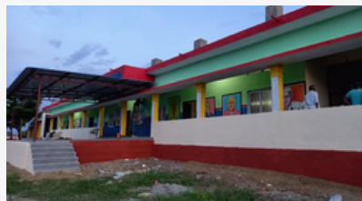
After classroom repair
